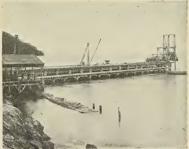
Dock Construction at the Port of Cristobal Colon, Venezuela. Reinforced Concrete, With Native Cement, is a Leading Factor of Present-Day Building Operations in the Republic
